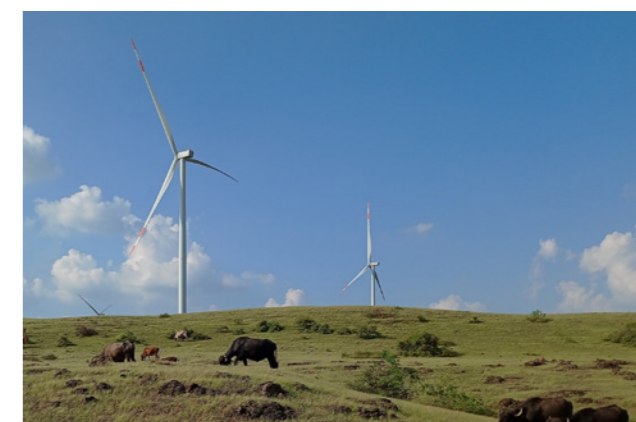
Kotada Pitha, Gujarat 16.2 MW wind | 9.8 MWp solar
