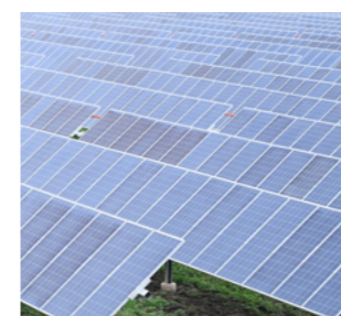
Akot, Maharashtra 14 MWp, Solar Farm
